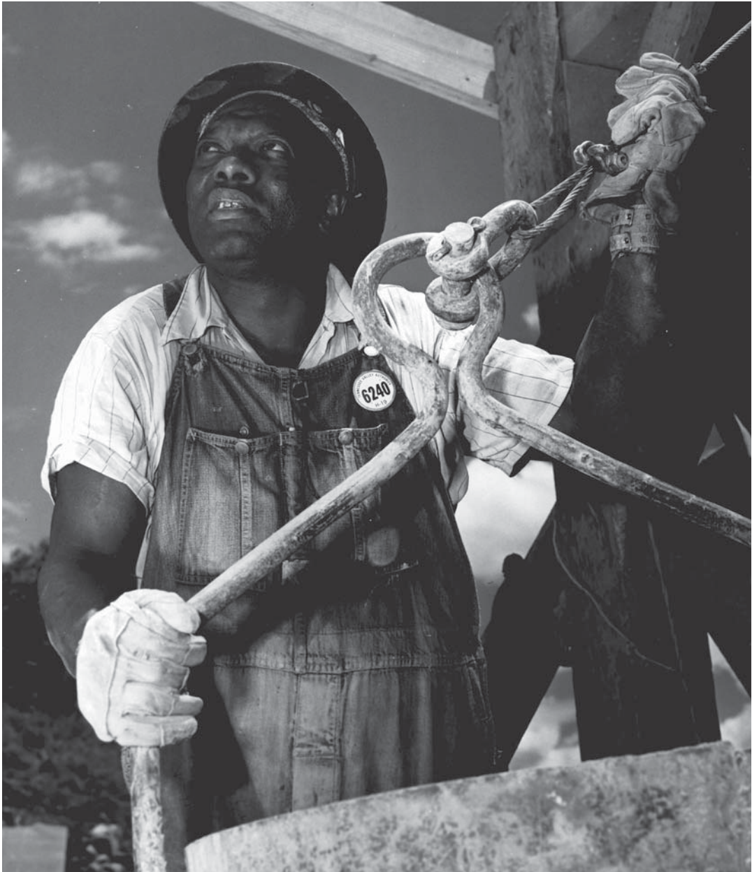
An African-American man working on construction of Douglas Dam in Tennessee, one of numerous Tennessee Valley Authority (TVA) projects. The TVA was one of the New Deal programs, which provided work to black and white laborers during the Great Depression.
